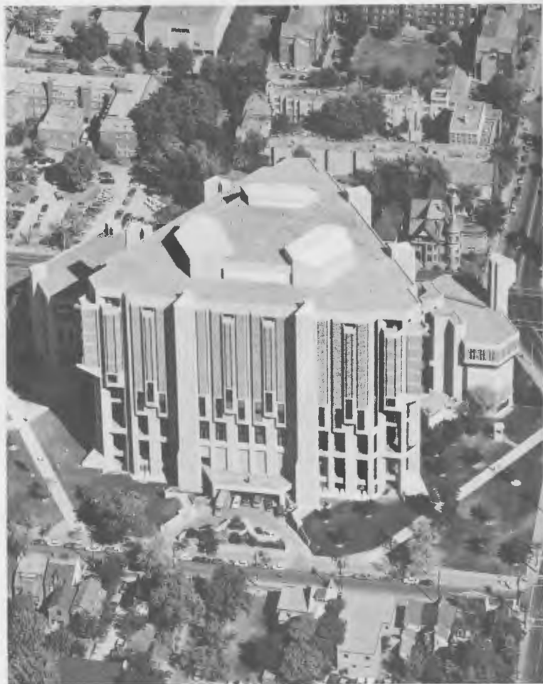
Aerial view of the John P. Robarts Research Library by the University of Toronto Zoology Media Services
