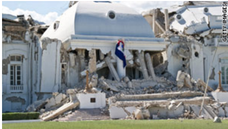
Buildings such as the presidential palace should have been built to higher standards, an OAS official says.
