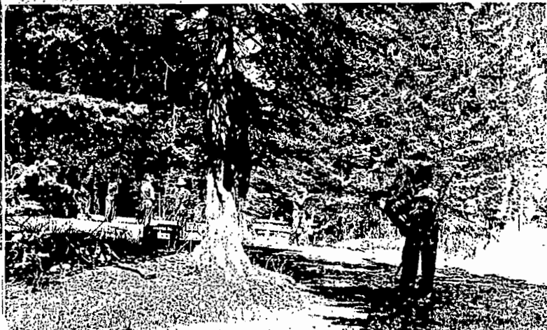
Improvement Work on Spire Rock Camp Ground
