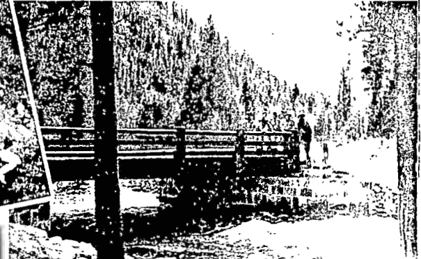
Trapper Creek Bridge
