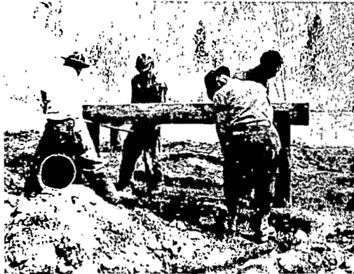
Putting Bench into Ground
