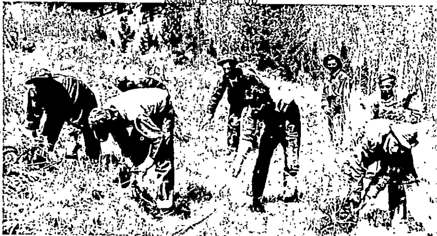
Clearing Side of Road
