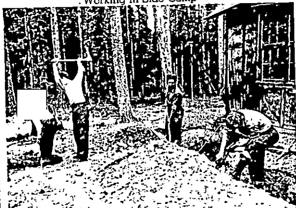
Work at Side Camp
