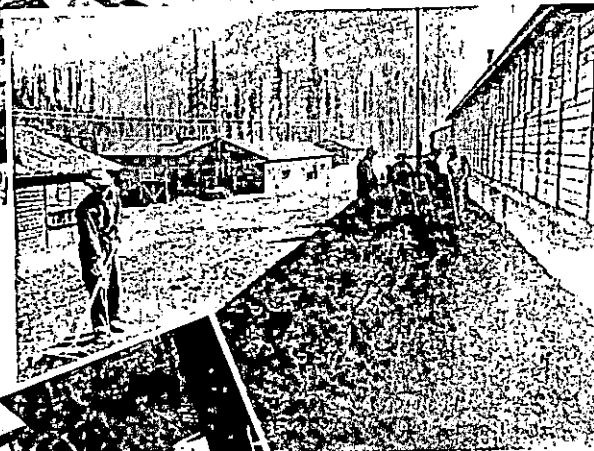
Working on Camp Area
