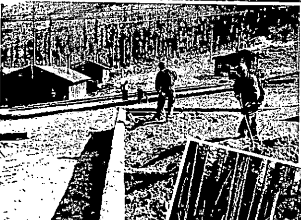
Working on Camp Area
