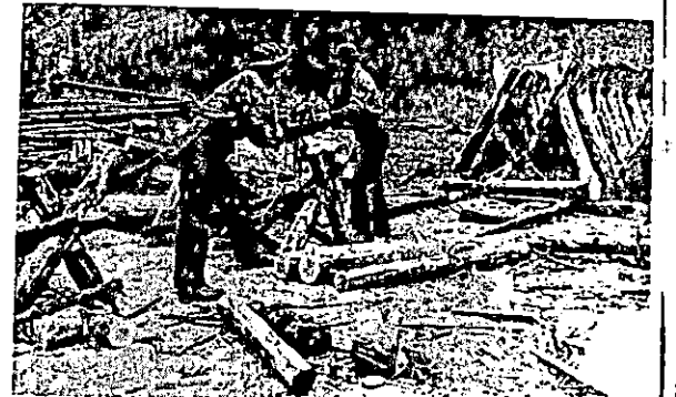
Peeling Poles, Sawing Lengths, and Stacking
