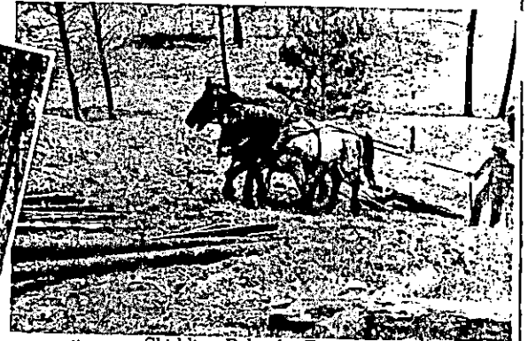
Skidding Poles for Fence
