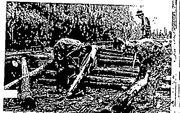
Peeling Poles, Sawing Lengths, and Stacking
