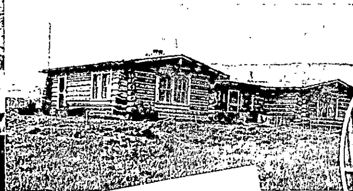
Foreman's House Constructed by CCC Boys (Side Camp No. 1)
