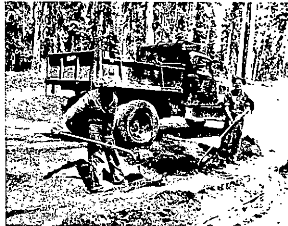
Sloping Road Banks
