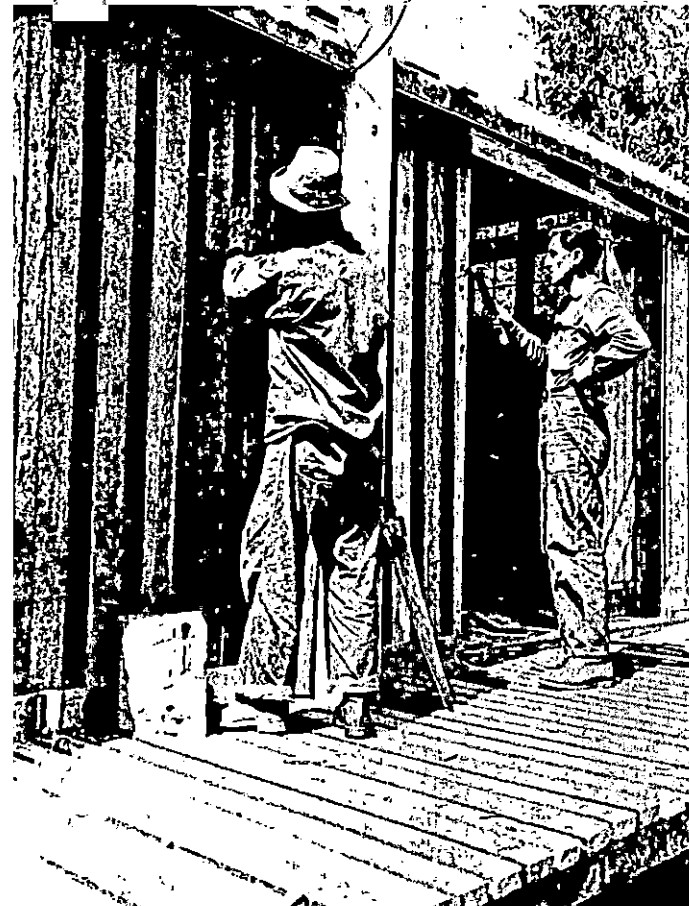
Constructing New Tool House
