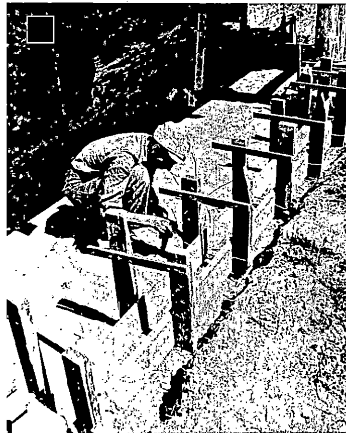
Making Cement Forms for Floor in Scout Building
