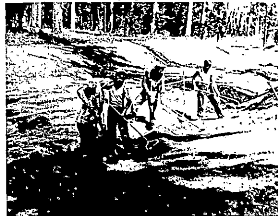
Sloping Road Banks
