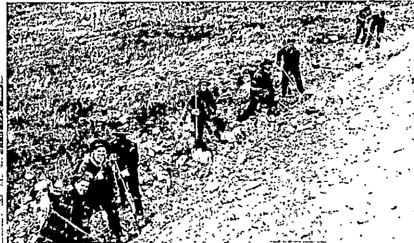
Work Crew Sloping Bank
