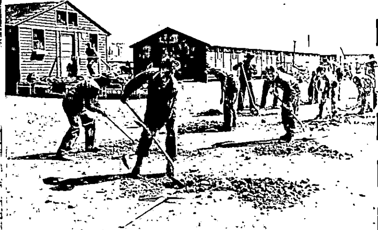
At Work Around Camp
