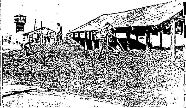
Working in Camp Area
