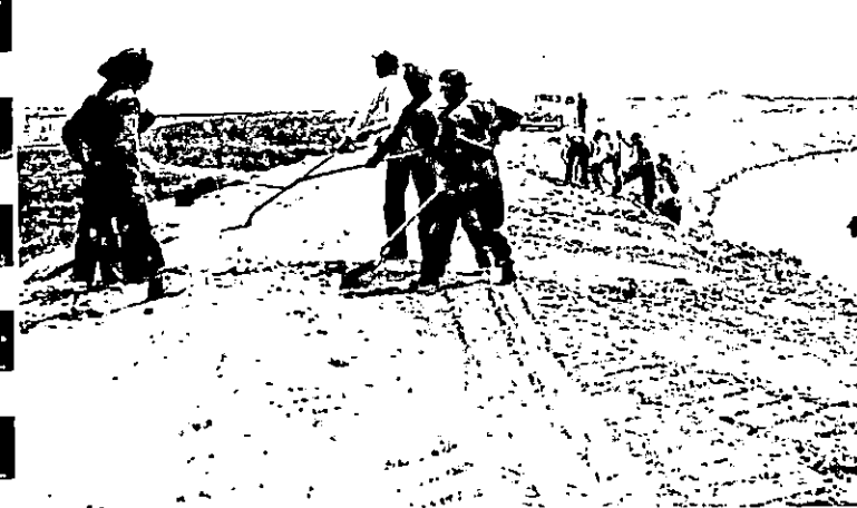
Lining Canal to Prevent Seepage
