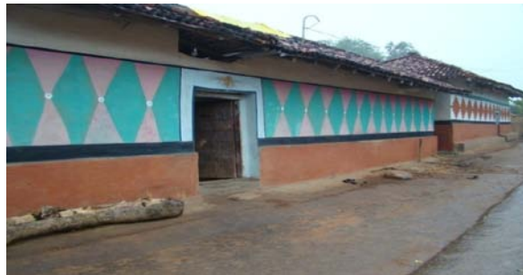
Fig. 5: Geometric shapes added within horizontal bands in Chauda village in Seraikela
