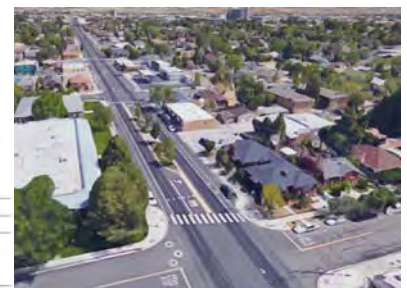
WELLS AVENUE IN RENO NV
